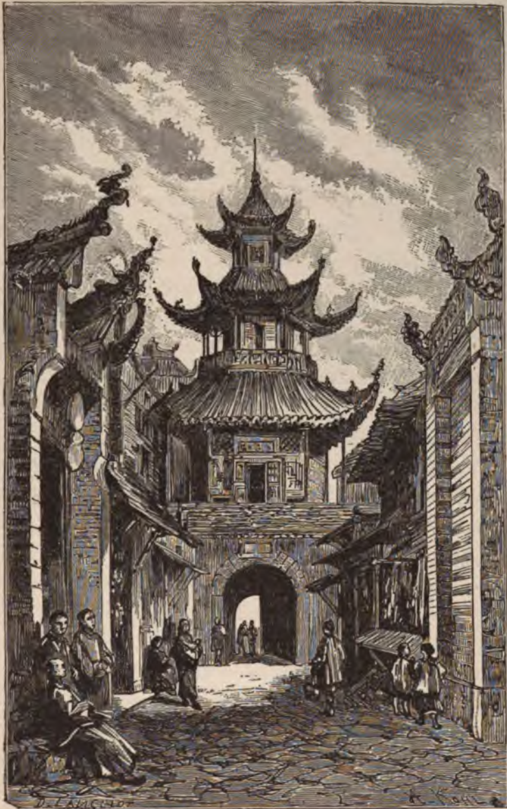
LOOKING THROUGH THE GATE.
